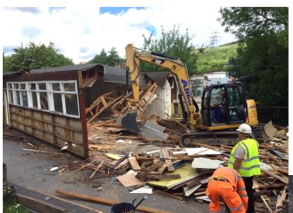
The photo shows the demolition of the old hut, the scale of the land released, area demolition of the works-side lobby, and the extent of the main church wall where underpinning is required.
