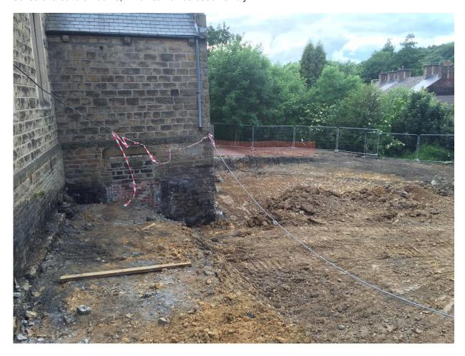
Part of the excavation work was to identify the full extent of the foundations of the existing church, and the requirements for underpinning. The excavations have revealed that there are no deep foundations along the north side of the church wall.
